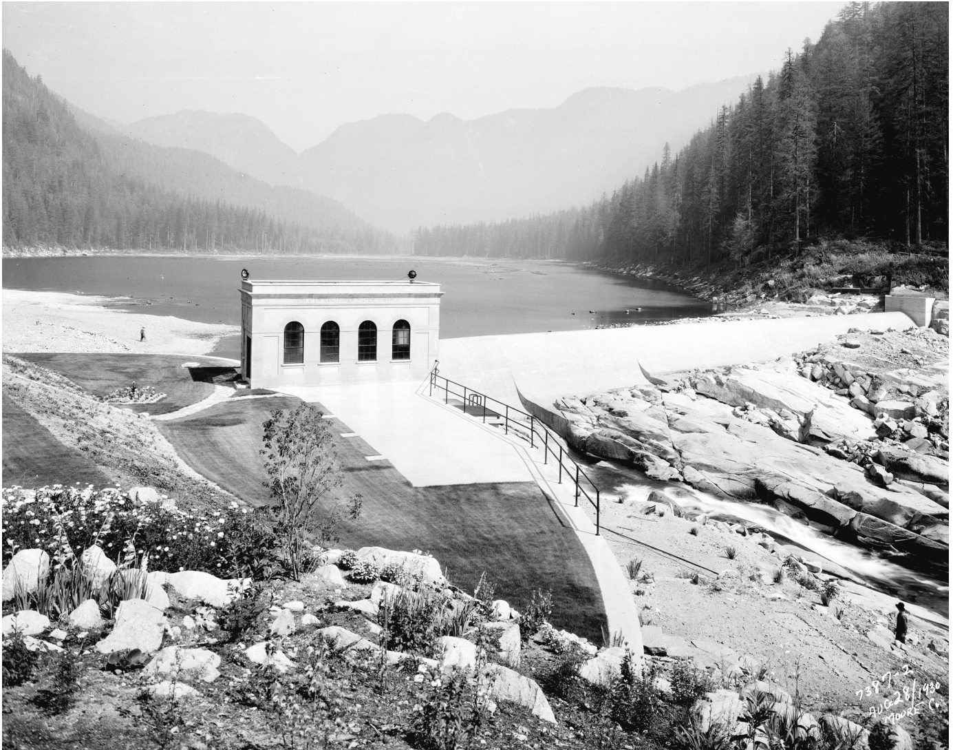
Figure 3: The dam at Seymour Falls was completed in 1926 and was crucial to transforming the river from being a natural waterbody with seasonal highs and lows into a reservoir tank that could be controlled to supply Vancouver with water. The building contained the screen house, through which the water passed before it was sent through a 60-inch, wooden conduit roughly four miles down the mountain to the city's distribution mains. The local grounds were also landscaped to improve their aesthetic appeal.
