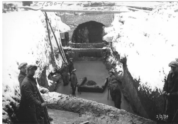
Figure 12.4 SEWER CONDUIT, MONTREAL, 1934
