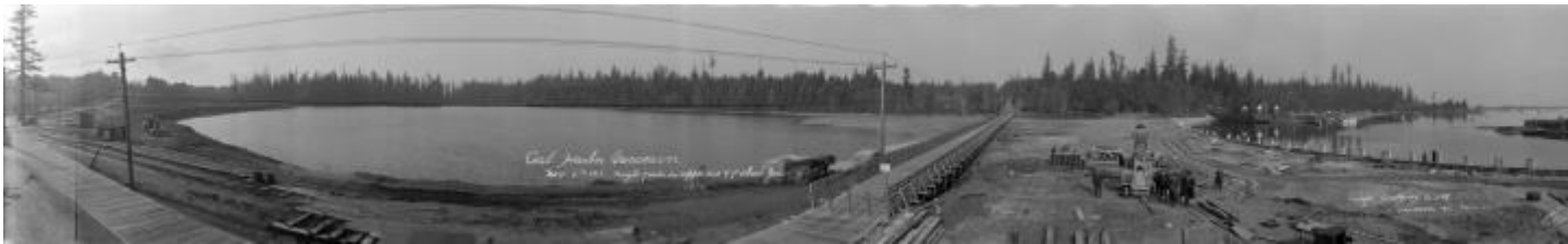
1.) Construction of Coal Harbour causeway, 1917. Source: City of Vancouver Archives, AM54-S4-3-: PAN N54.
