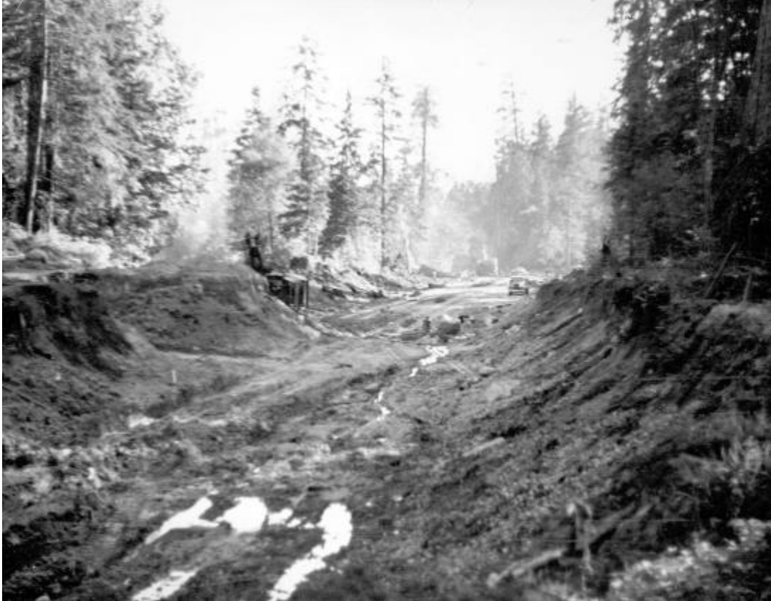
2.) Cutting the road to Lions Gate Bridge, 1937. Source: City of Vancouver Archives, AM54-S9-: CVA 265-14 .
