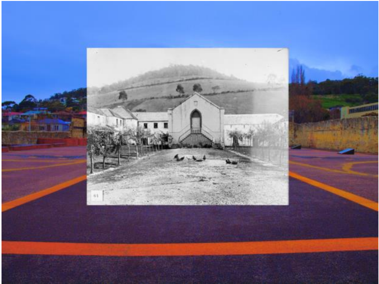
NS1013-1-1757 The Chapel, Cascades Factory (Women's Prison). Tasmanian Archive and Heritage Office.
