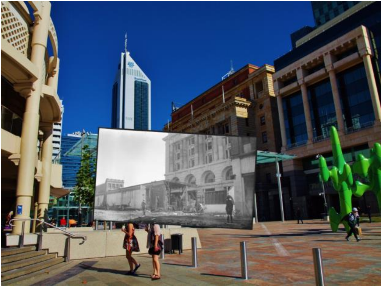
State Library of Western Australia 304413PD, Demolition of buildings next to General Post Office.
