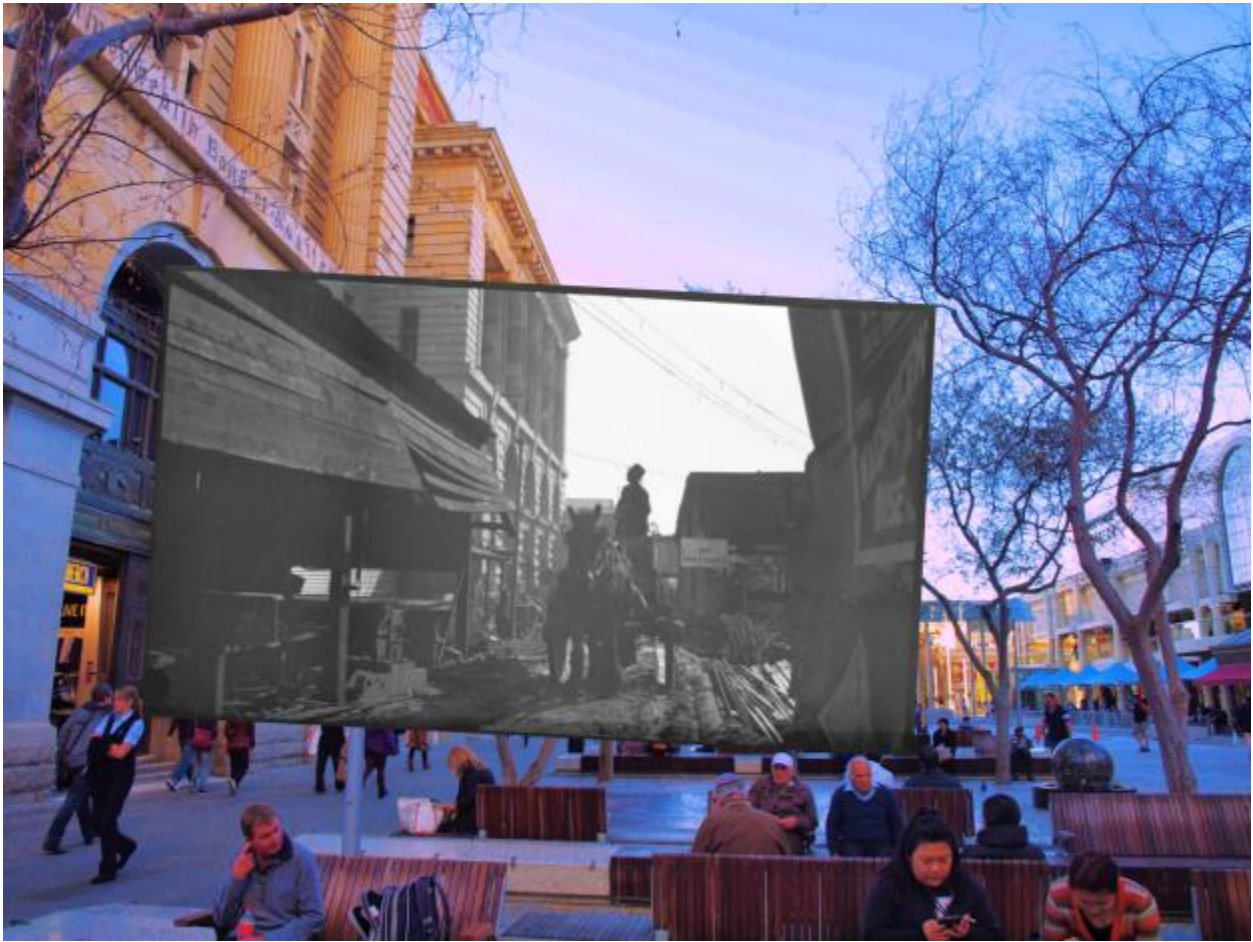
State Library of Western Australia 304412PD, Demolition of buildings next to General Post Office.
